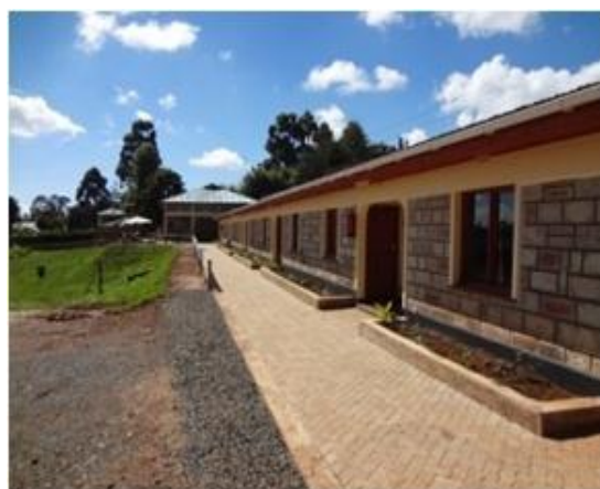
Figura 8 Vista externa hospedaje (HACT). Fuente: High Altitude Training Centre – Iten (2017).
